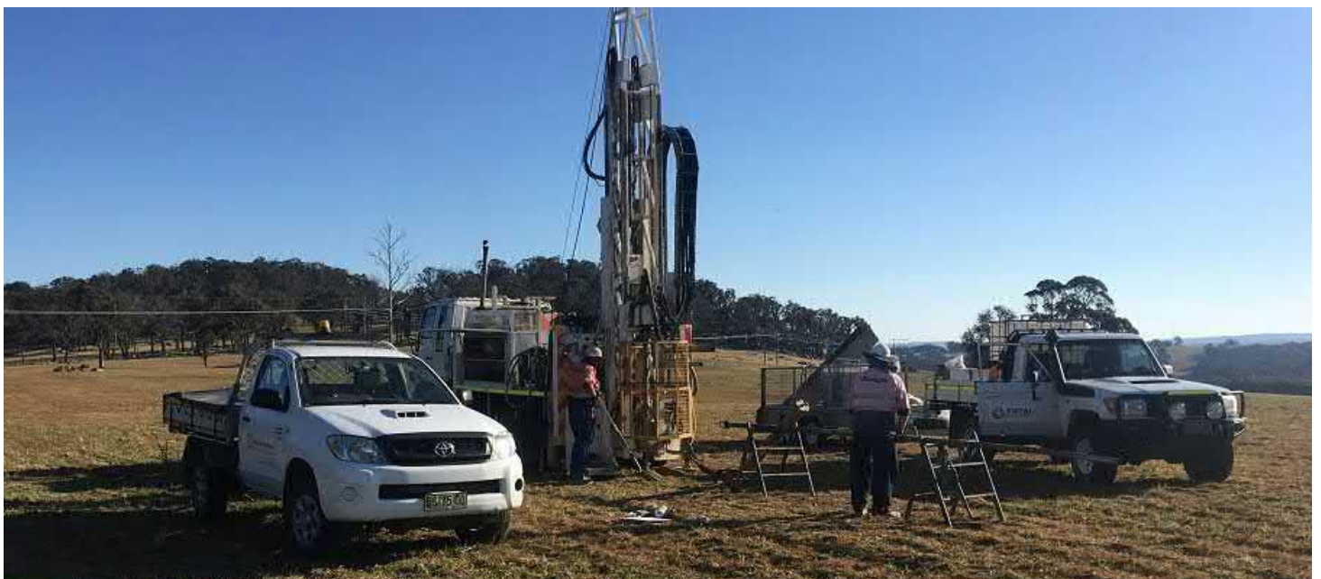
Fig 2: Typical setup for a geotechnical investigation
